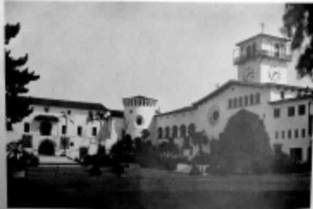
Santa Barbara County Court House, Santa Barbara, California, William Bruce Company, architect
